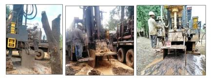
been drilled and four dry wells were drilled. The Hawassa Water Bureau (WB) has agreed to provide four additional new sites to replace these. The Water Bureau has also required us to drill 8 inch bore holes and pack gravel around the 4 inch casing for all future wells. This adds
