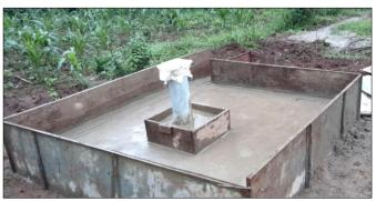
Left: Gashaw standing with the school director and other staff members at the well site. Center: Mixing the cement with volcanic rock and sand for the pump pad. Right: The completed installation is ready for the pump to be installed as soon as the cement is dry.
